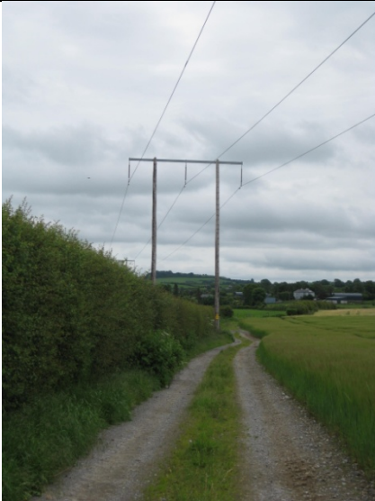
Plate 3: IMP82, looking SE.
