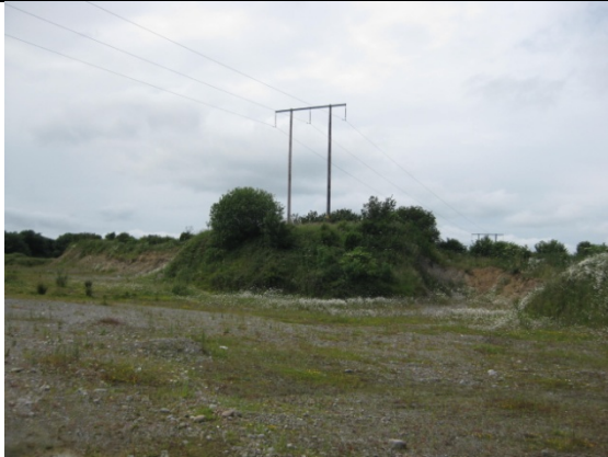
Plate 7: IMP89 at edge of quarry, looking NW.
