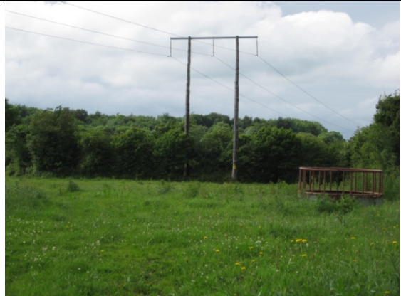
Plate 10: IMP93, looking NW.
