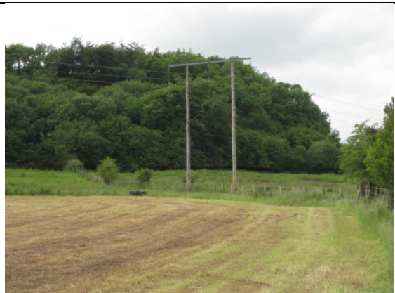
Plate 12: IMP95, looking NW.
