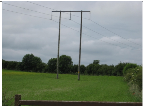
Plate 6: IMP88, looking NW.
