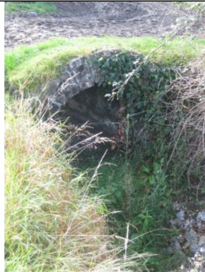
Plate 6: Stone culvert at stream crossing between BC3 and 4.
