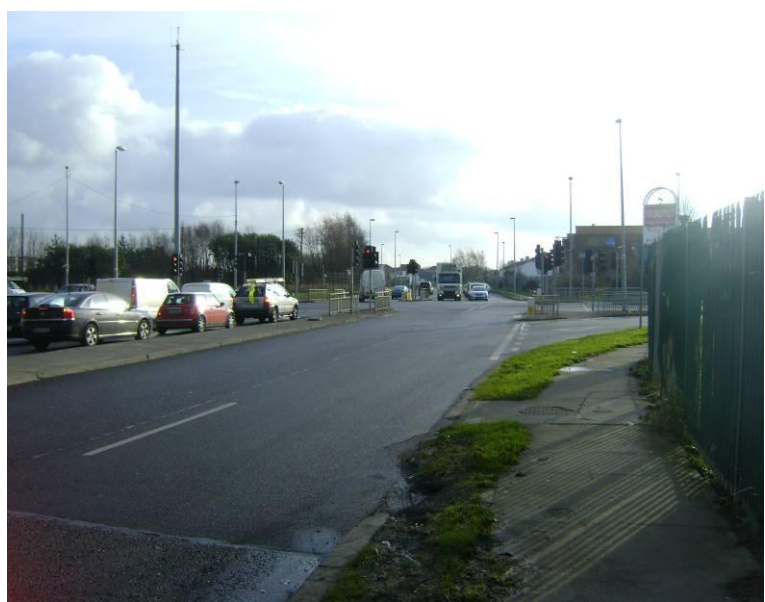
Photo 2.7: Looking east along R139 towards exit of Clarehall Junction
