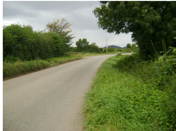
Photo 2: R426 looking north towards site access
