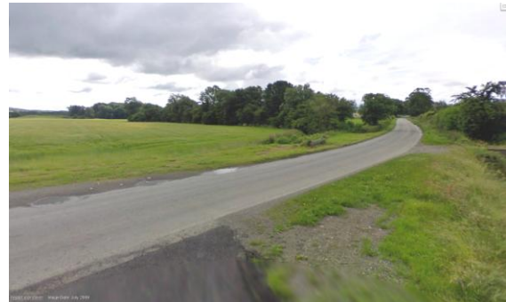
Photo 2: R426 looking South opposite site
