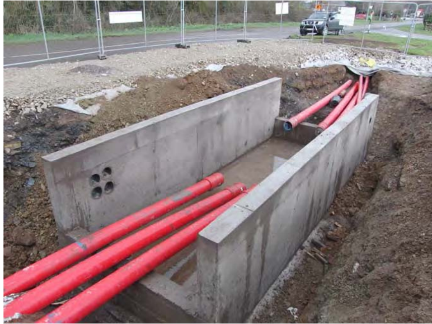
Figure 2: Typical Joint Bay Construction Adjacent to Public Road
