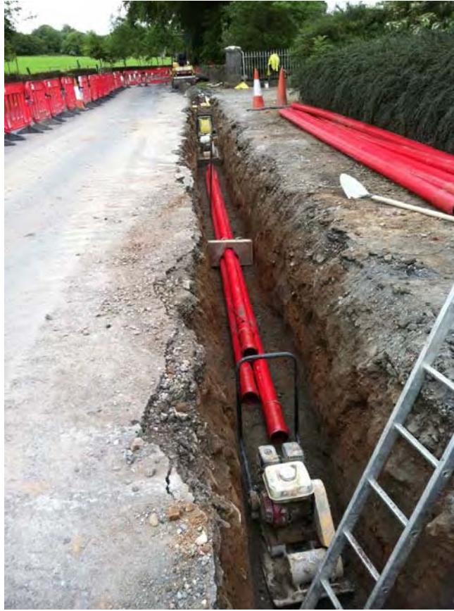
Figure 1 : Typical 110kV Trench Excavation (Ducts in Trefoil Formation)
