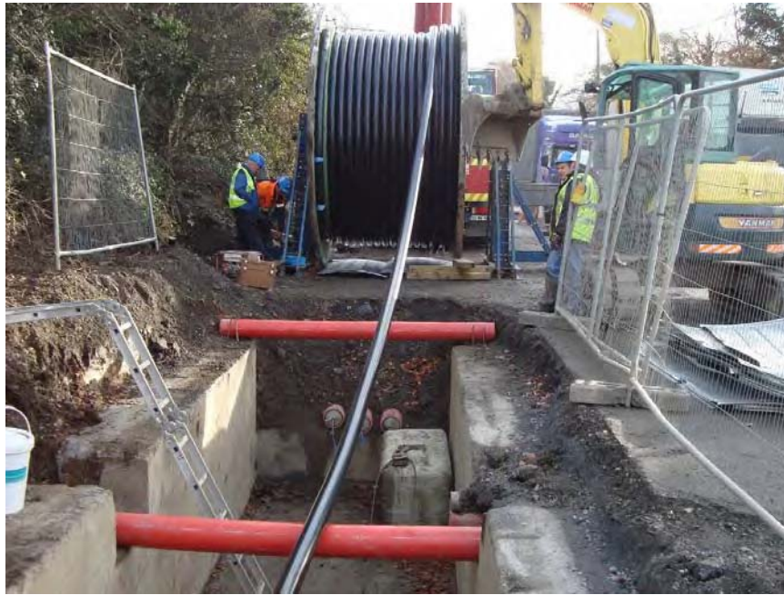
Figure 3: Typical HV Cable Installation
