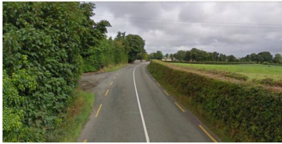
Photo 1: R432 Looking North
